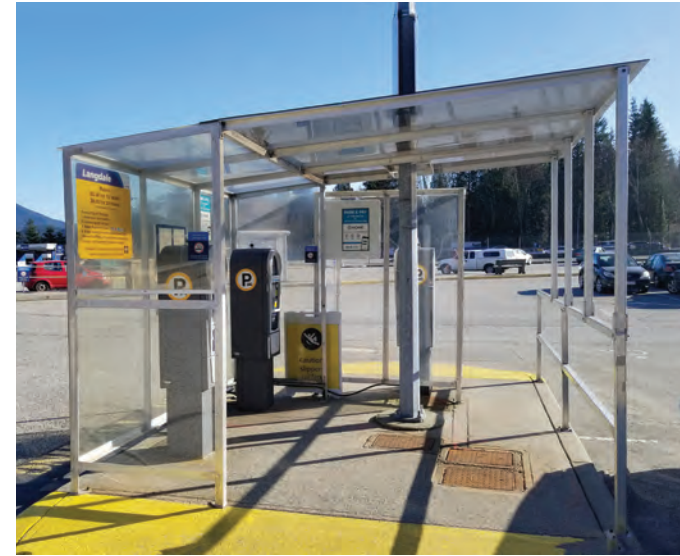
The new extended cover over the parking lot ticket machines.
