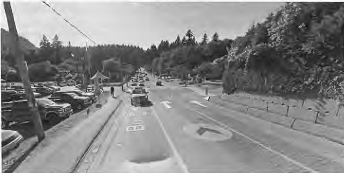
FIGURE 3 Bowen Island Trunk Road at Cardena Road Intersection
