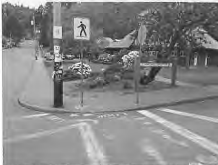
Photo 9 - Northwest Corner Bowen Island Trunk Road & Cardena Road
